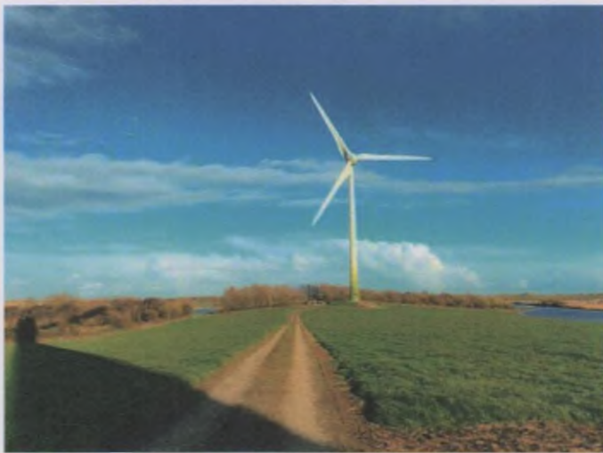
Plate 13: T16 and associated access road, looking ENE.
