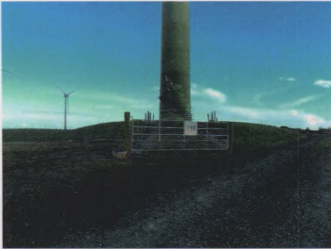
Plate 15: T18, looking SE.
