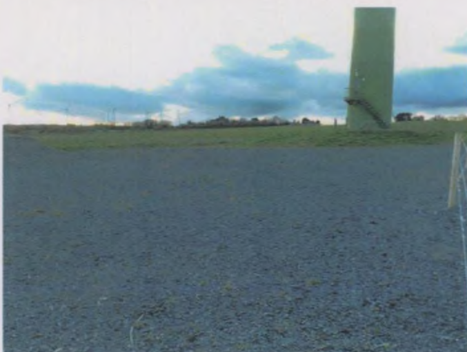
Plate 20: T23 and associated hardstand.
