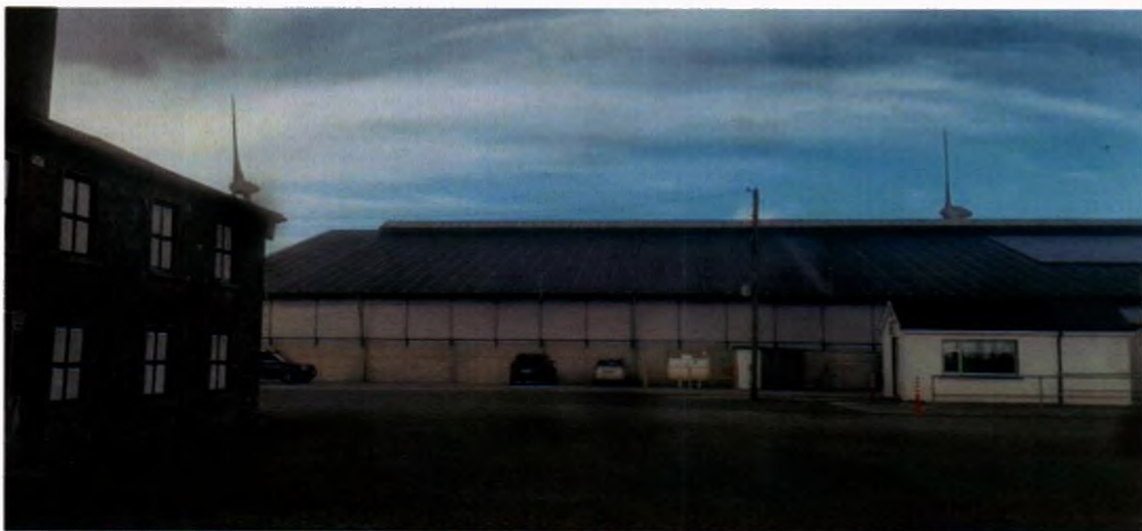
Plate 4-2 South facing aspect of Ballywater Dairy Farm (west side).
