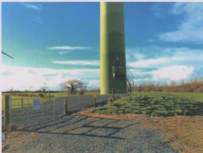
Plate 7: T10 and associated hardstand, looking WNW.
