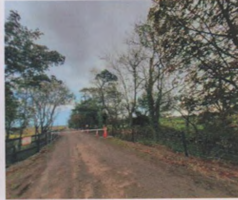
Plate 4-20 Main site entrance to southern side of wind farm with broadleaf species treelines.
