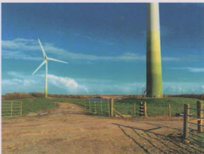
Plate 14: T17 looking SE.
