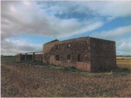
Plate 4-7 East facing aspect of the PRF.
