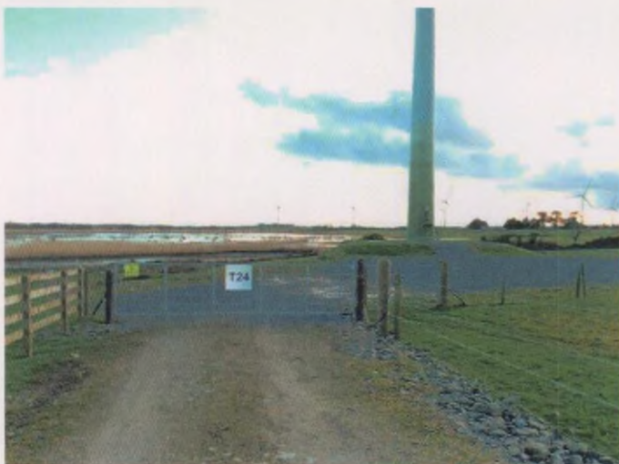
Plate 21: T24 and associated hardstand, looking SSW.
