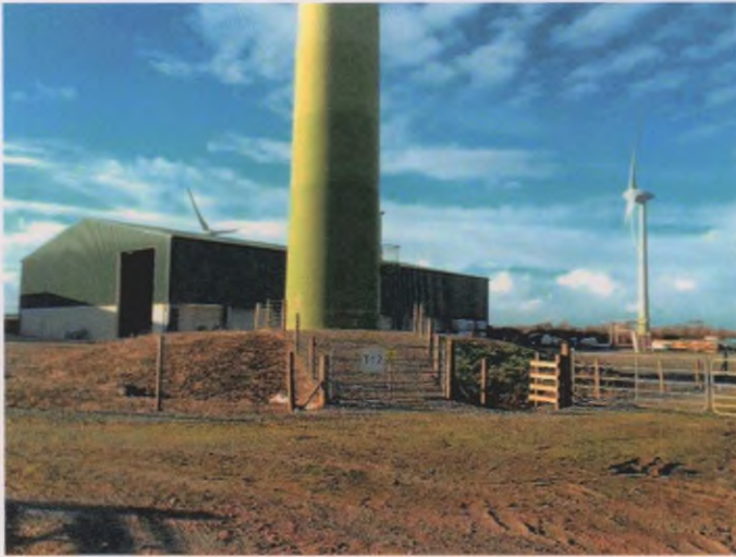
Plate 9: T12, looking NW.
