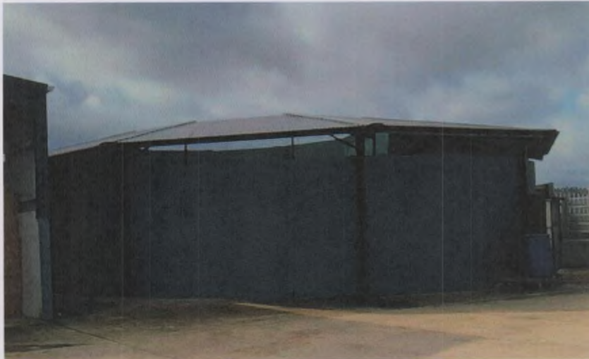
Plate 4-15 North-east facing aspect of the horse walker.
