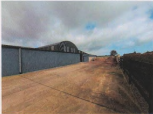
Plate 4-9 East facing aspect of the stables.
