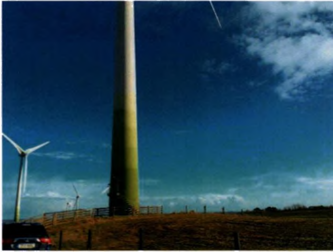
Plate 1: T3, looking SE.
